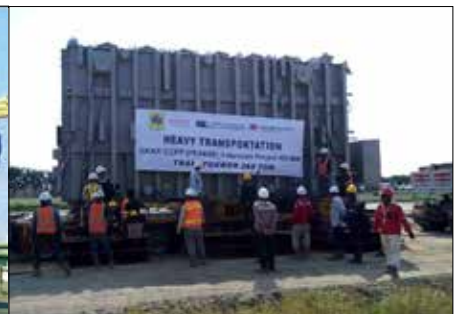
TRANSFORMER Transportation (LxWxH @ 11.8X4.4X5.5 M/288 TON)
