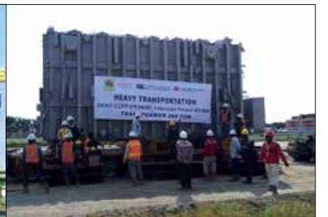
TRANSFORMER Transportation (LxWxH @ 11.8X4.4X5.5 M/288 TON)
