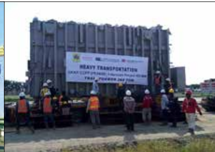
TRANSFORMER Transportation (LxWxH @ 11.8X4.4X5.5 M/288 TON)
