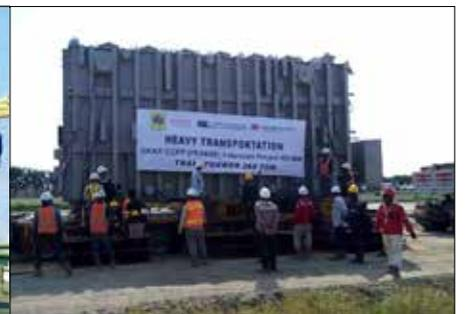
TRANSFORMER Transportation (LxWxH @ 11.8X4.4X5.5 M/288 TON)
